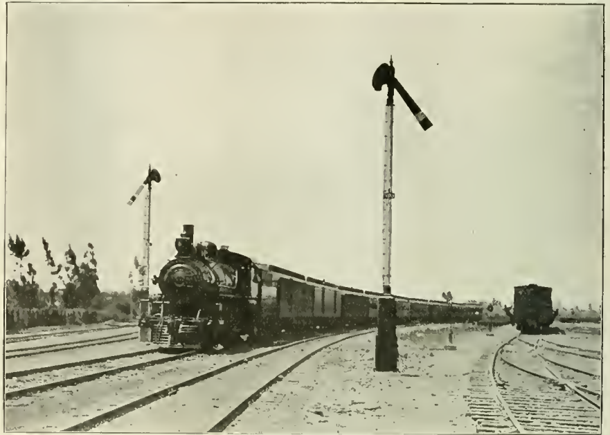
SOUTHERN PACIFIC ROAD NEAR SAN JOSE, CAL.
